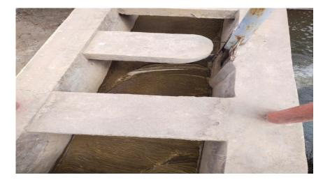
3) **Flocculation:-** Flocculation is a process by which a chemical coagulant added to the water acts to facilitate bonding between particles, creating larger aggregates which are easier to separate. The method is widely used in water treatment plants and can also be applied to sample processing for monitoring applications.
