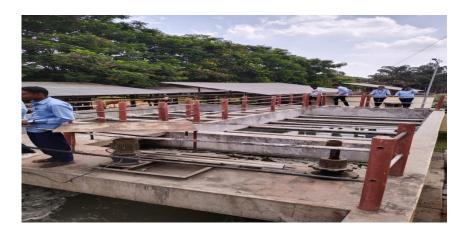
4) Sedimentation:- is the process of allowing particles in suspension in water to settle out of the suspension under the effect of gravity. The particles that settle out from the suspension become sediment, and in water treatment is known as sludge
